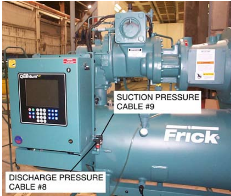
Figure 18a. Wiring Harness Installation, RXF 24 — 50.
